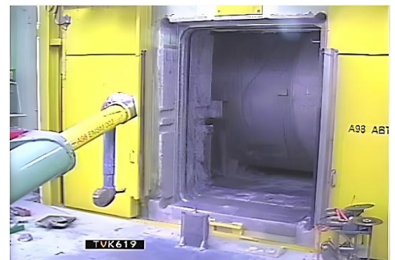
View on the HAWC storage tank
